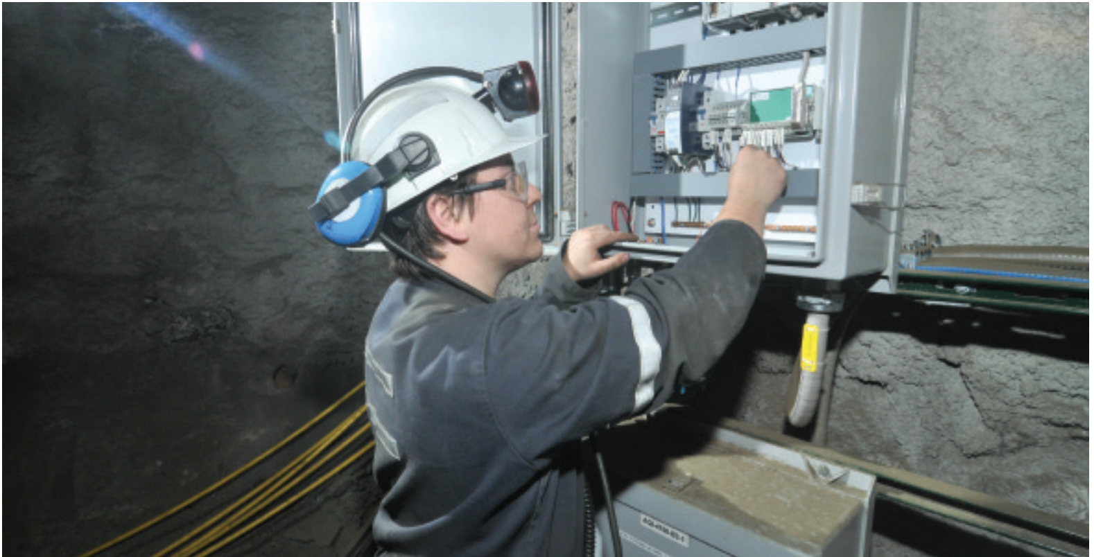
Paul Lalonde, Bestech automation specialist, reviews air quality instrumentation control point that collects data from the environmental monitoring sensors at Coleman Mine.
